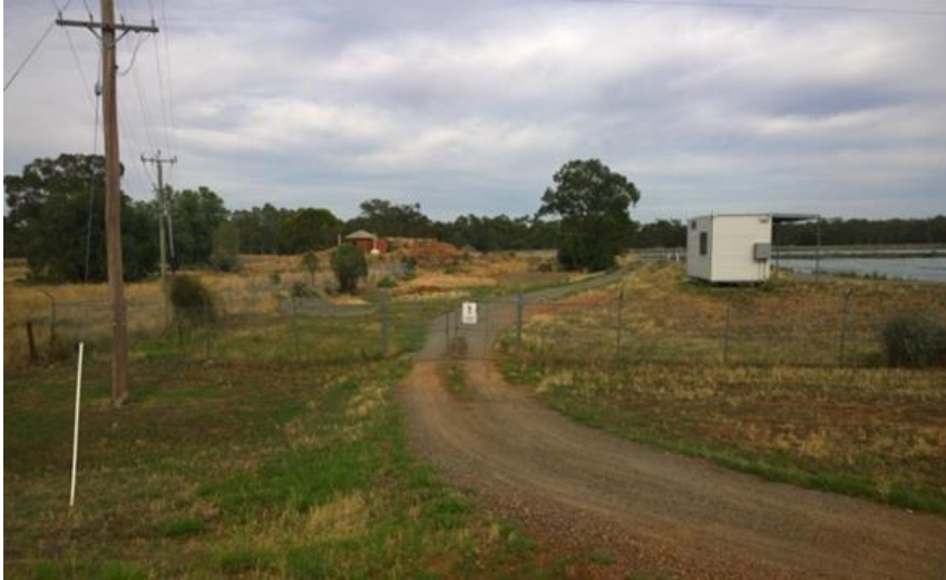
Figure 4 – Nyngan Sewage Treatment Plant
