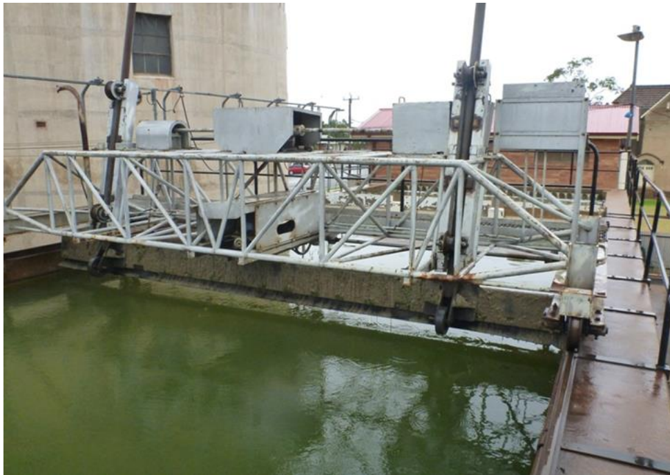
Figure 2 – Nyngan Water Treatment Plant Sedimentation Tank
