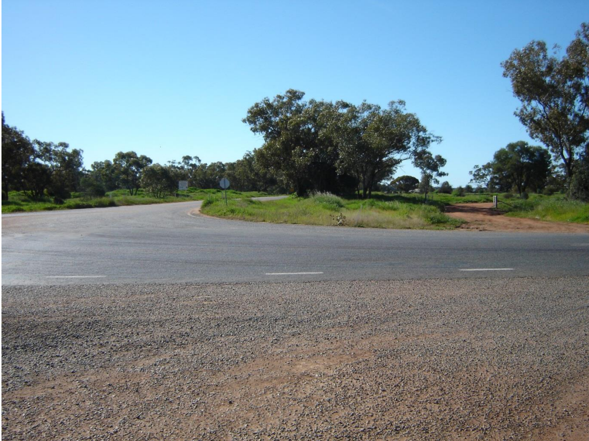
Property Access onto Barrier Highway adjacent to Yarrandale Road Intersection.
