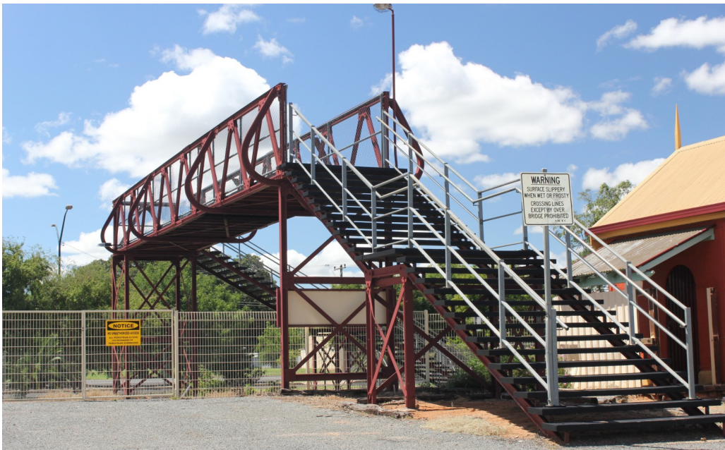
Railway Pedestrian Bridge
