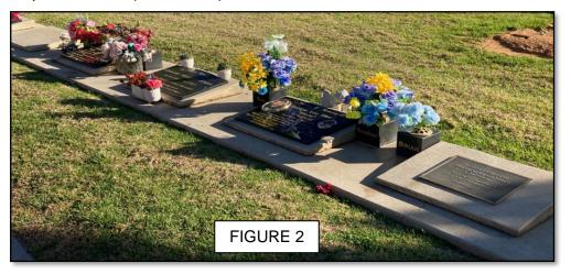
Staff have suggested replicating this approach for the new section of the lawn cemetery, using individual precast concrete headstones that are poured off site and placed as required. These headstones can then have a brass or marble plaque fitted to the concrete as with the existing lawn and ashes sections.
