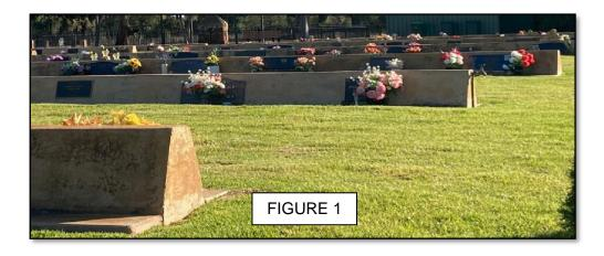
The current formwork is old and damaged and requires replacement. This formwork is expensive to replace, it is difficult to handle, and requires a lot of concrete and labour to construct a strip of headwall which results in significant cost to produce this style of headwall.
